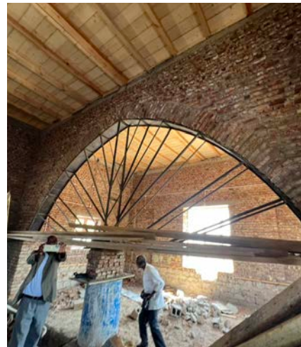
Interior Arch – Timber and concrete roof.
